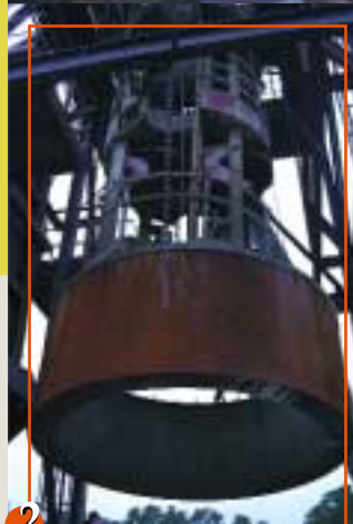
Picture 2: Installation of the first prefabricated reinforced concrete rings
